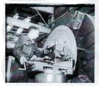
The photo here shows Len Berghoff on the Craven lathe turning the air grooves in a scavenger valve disk. These are made of aluminium, and after he has finished the turning operation they will be cut into segments. This is a delicate process, for one time he had a 'dig' in with the tool and the whole assemble shattered to pieces. Fortunately Len did not suffer any ill effects as the pieces fell into the bed of the machine.
