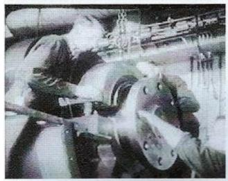
The fitting of one of the main bedplate bearings is shown here. My brother Raeburn who commenced his time in 1948 is shown helping fitter Bert Woods with the aid of the overhead crane and Joe Costello, the rigger, who is signalling the crane driver approximately 60 feet above, to aligning the keep before bolting home. Lead wires are placed between the keep and the shaft, flange of which is shown, bolted down, removed and measured with a micrometer to obtain correct clearance. If this is
