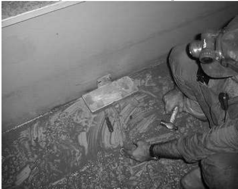
Figure A.1: Installation of Tsevas Pitguard
