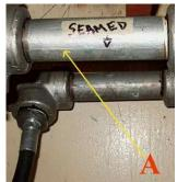
The amateurish installation of some of these nipples via excessive force has caused significant damage to them. These bite marks from the pipe wrench used, penetrate the sidewall of the pipe,
