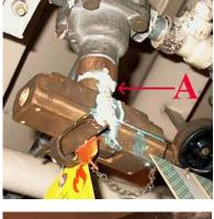
The bracketing used to support the new installation is rather lightweight given the magnitude of the shock loading that can occur upon deployment of the CO<sup>2</sup> gas. In the picture at the right, one can see that this particular bracket is only tacked on to the support steel as denoted by the green arrow "A". Failure is certain to occur at this location. These brackets should be replaced with units of heavier construction.
