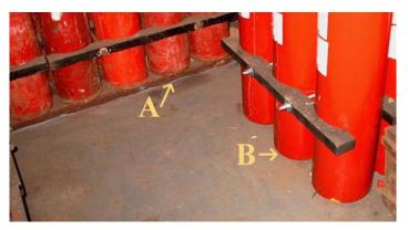
indicated by "A", while "B" shows direct mounting on the steel deck. The lower picture shows the entire bank of new cylinders in the paint locker on the steel deck.
