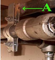
These pictures illustrate a shortcut taken in the installation of the extra cylinders. It is common practice to mount cylinders on a wooden base if a steel deck is present. This is to prevent fretting of the base of the cylinders induced by vibrations from normal ship operations, which can therefore weaken a cylinder, risking potential failure of said cylinder. The picture at the right shows the wooden base below cylinders as
