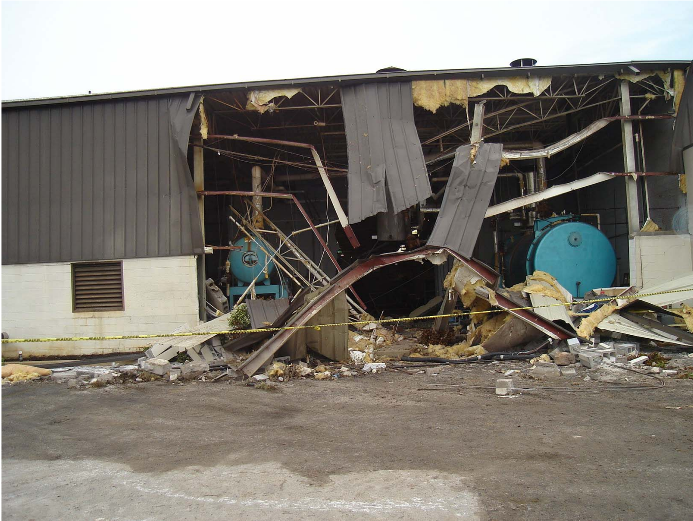
Photo #6 – View of East Wall from Outside Plant
