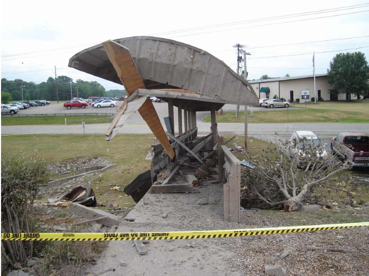
Photo #8 – View of Pedestrian Walkway Bridge
