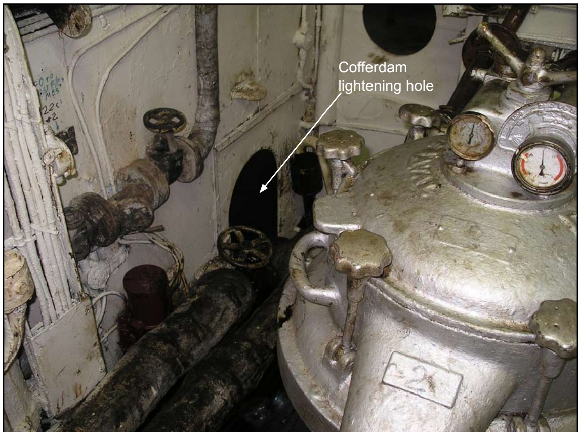
Entrance to the cofferdam (view from the purifier room)
