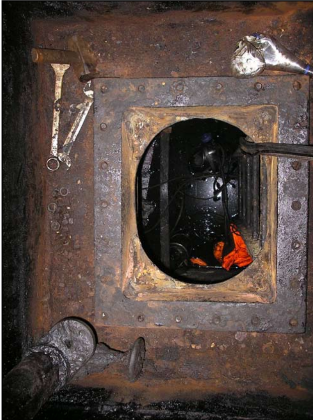
No.4 port outer double bottom tank manhole
