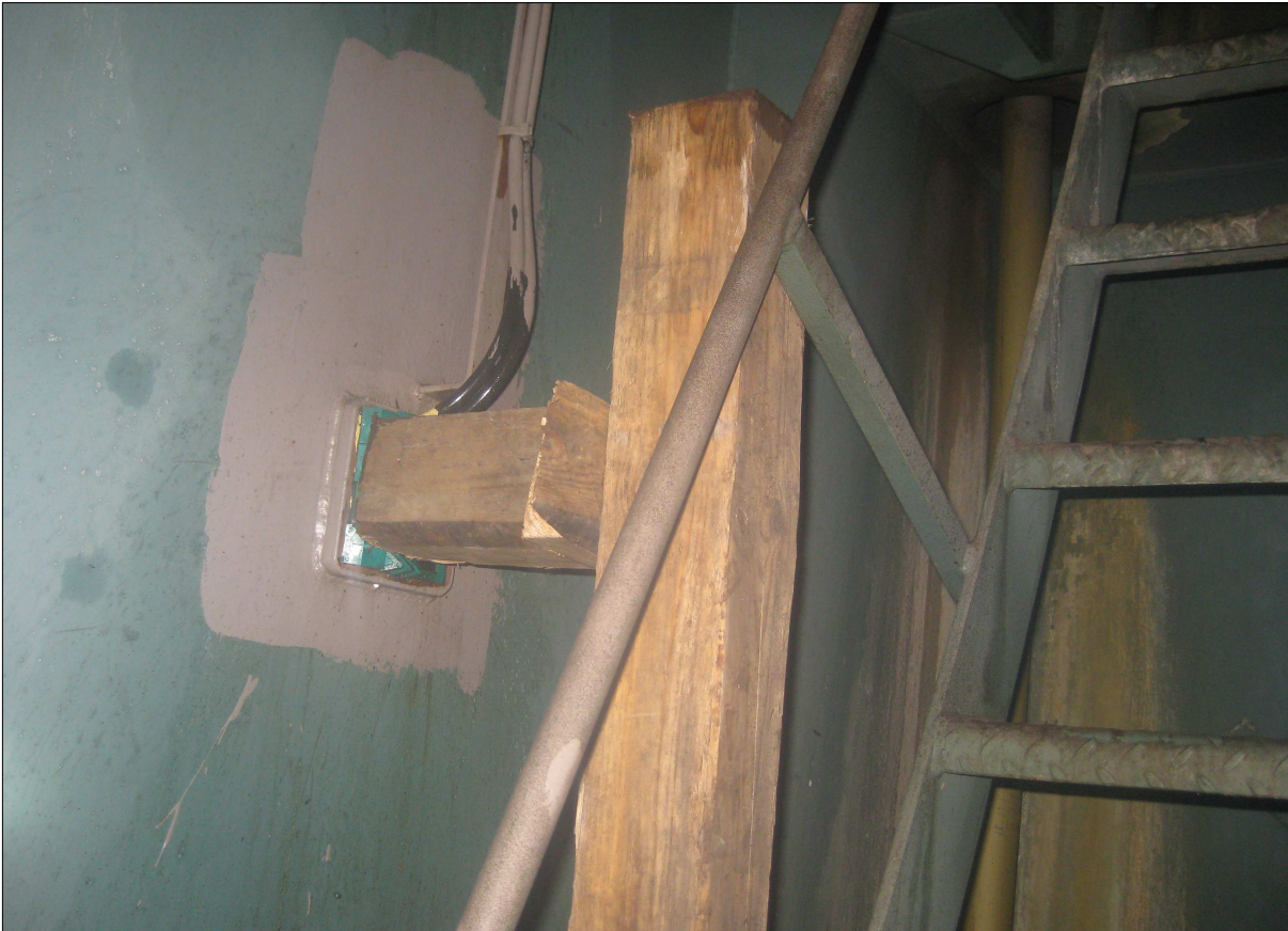
Figure 25: Temporary repair of cable penetration in bulkhead between emergency exit and cargo hold Source: Maersk Line
