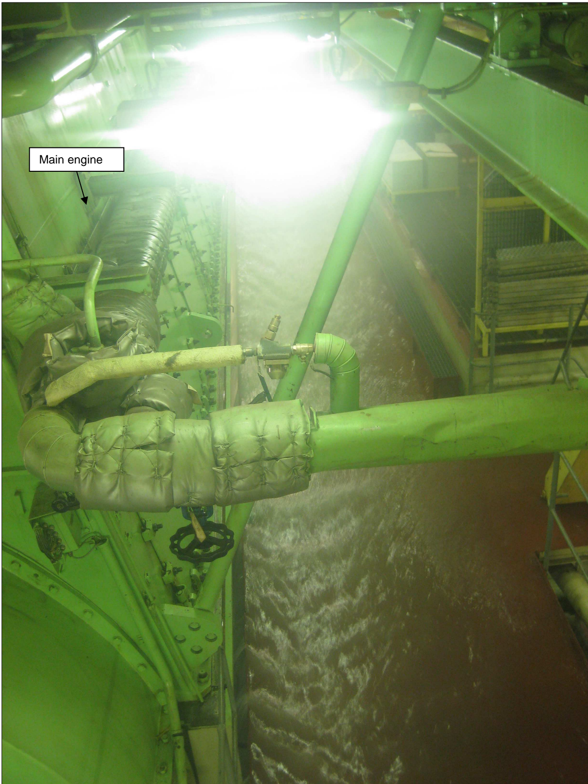
Figure 21: Engine room getting flooded Source: Maersk Line
