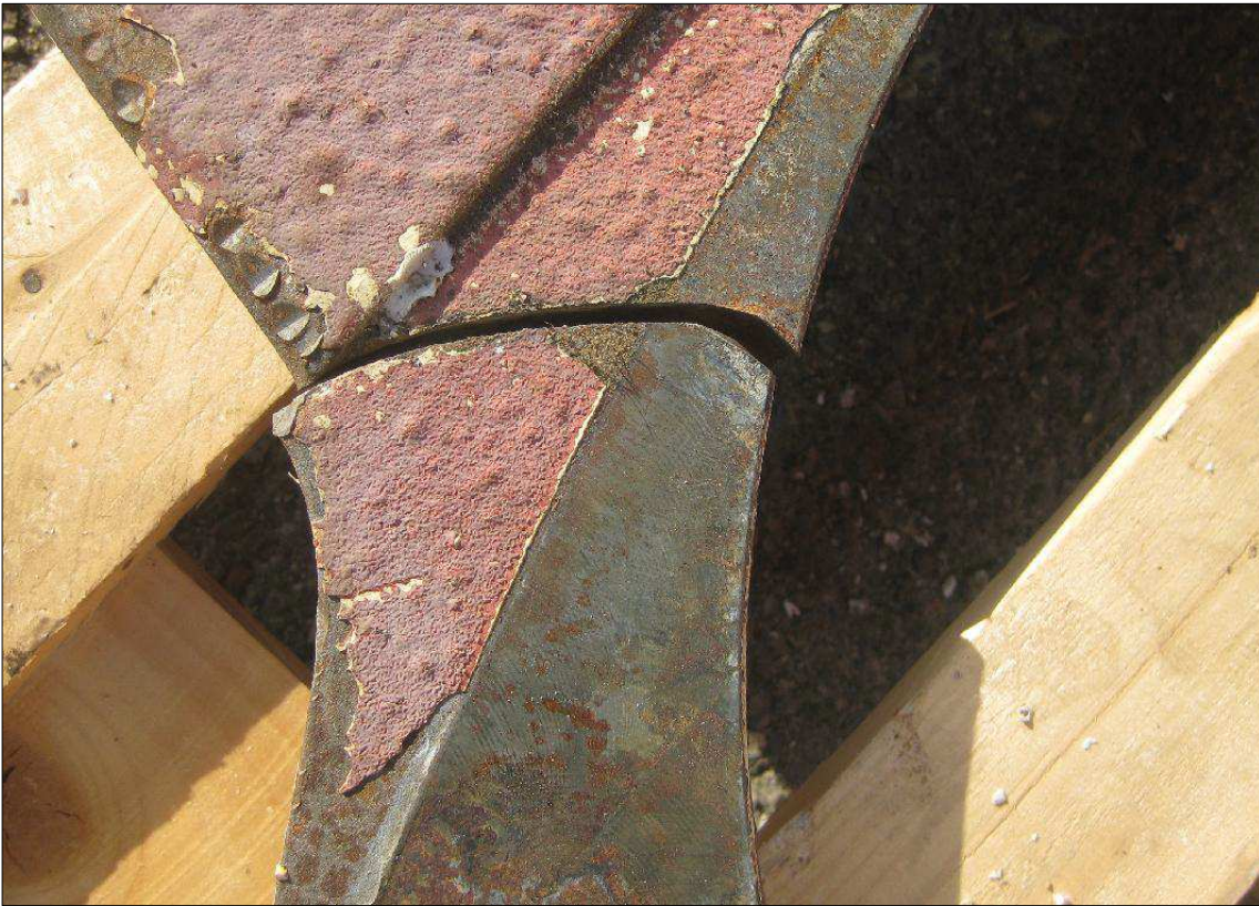
Figure 55: Fracture of supporting base plate for the aft stern thruster Source: BANDAK Engineering/Rolls Royce Marine
