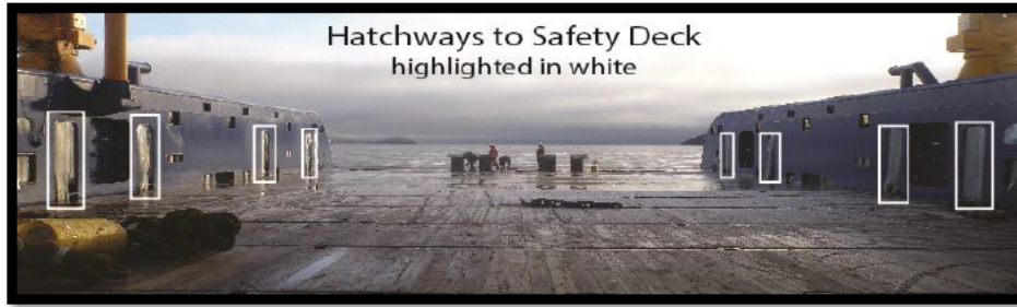
Figure 69: Photo depicting location of hatchways into safety deck from aft working deck of AIVIQ. (USCG Photo and Developed)
