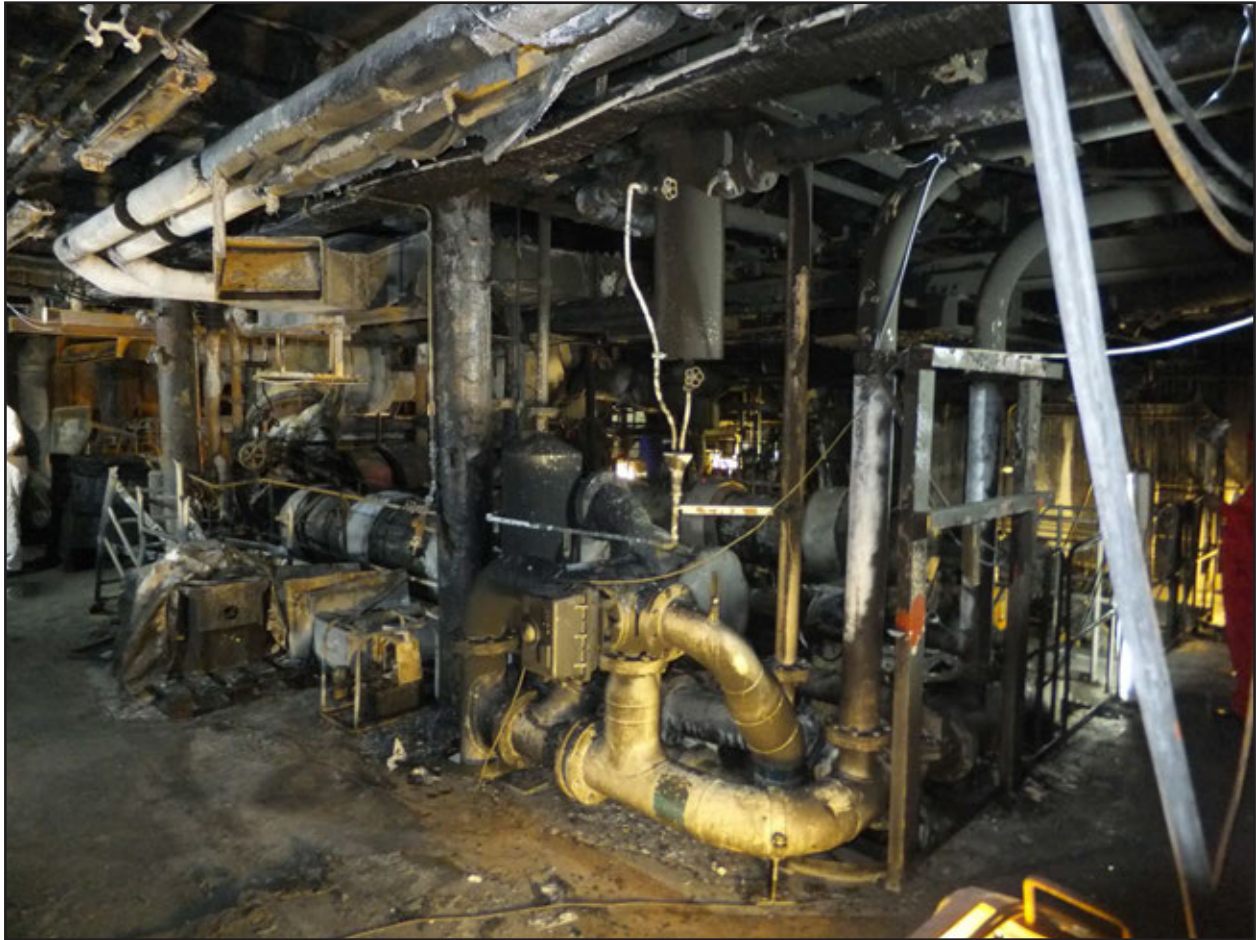
Figure 10: Fire damage around starboard main engines, deck 2
