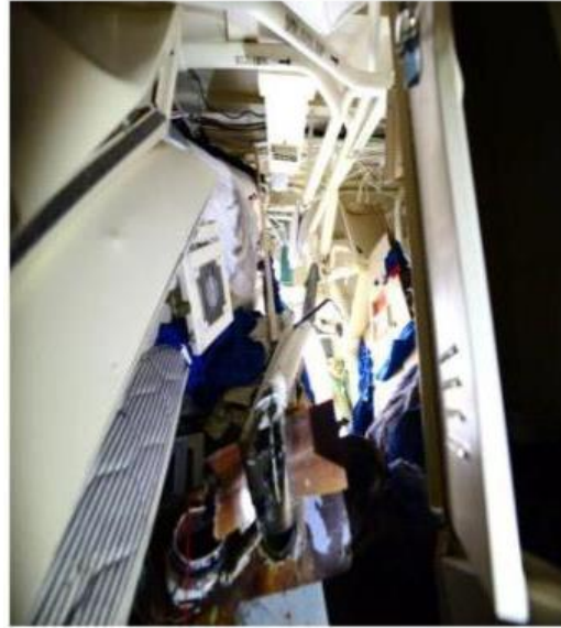
Figure 16 – Berthing 3 facing port after collision
