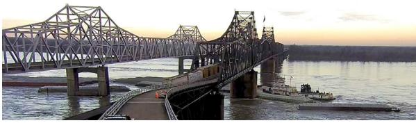
**Figure 59.** Barges broke away from the *Chad Pregracke* after the tow struck pier 3 of the Old Highway 80 bridge. Source: COAST GUARD.
