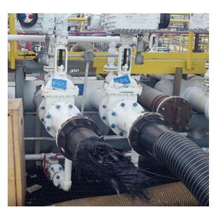
**Figure 24.** Damaged shoreside cargo hose and deformed piping at the manifold at the Kinder Morgan facility.
