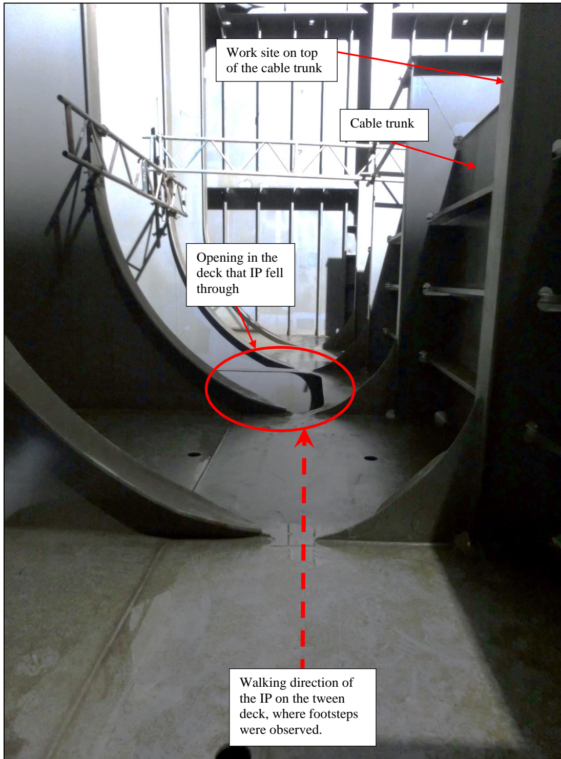
Figure 12: Access ladder passing cable trunk. Lighting conditions are similar to those at the time of the accident
