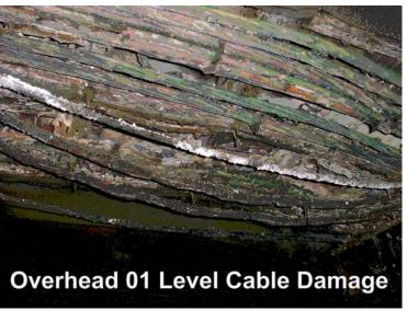
Generally all lighting, annunciating and visible alarms, shields and lense covers were destroyed on this level (01) and the next upper level in this space (02). The paint on various equipment, structures, and pipe lagging or coverings was damaged on the upper levels. Two large intake plenums above the port main engines were warped because of the fire. In the same general area and damaged after closing were actuating cylinders that operated the inlet dampers for exhaust fans of this space.
