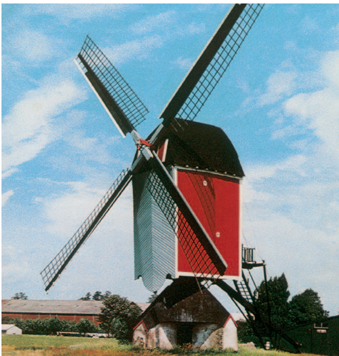
Fig. 1: The windmill – ancestor of the axial turbine. This type has been in use since the 13 th century.
