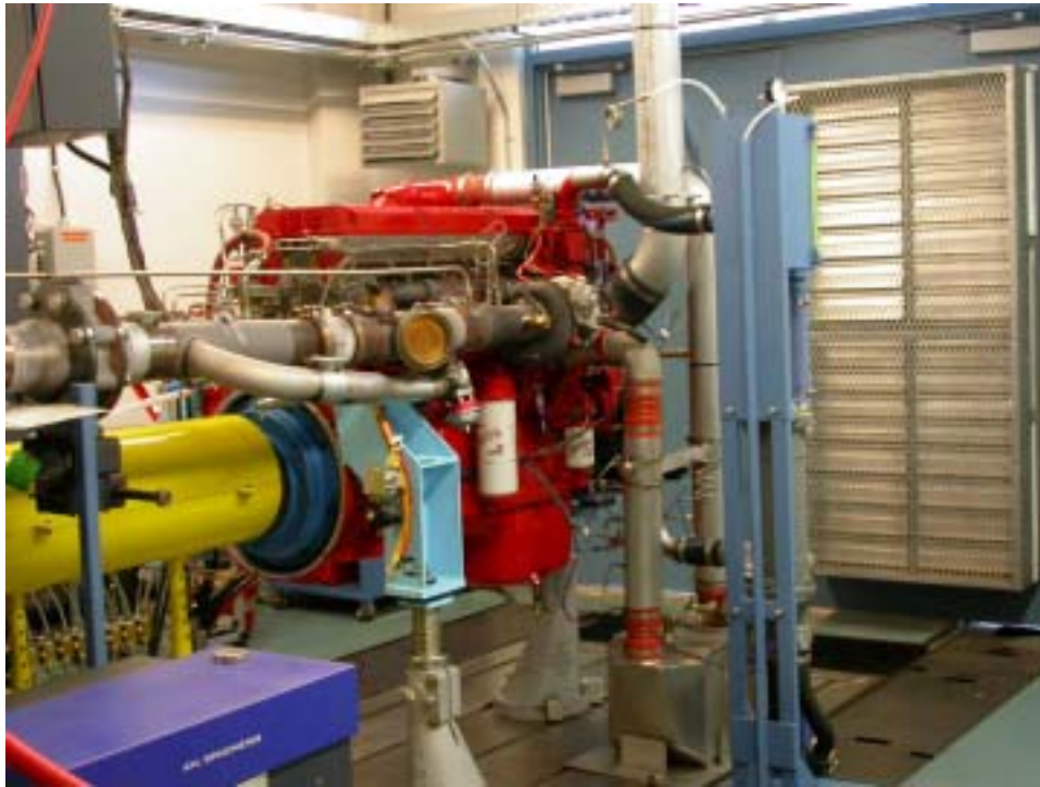
Figure 49: New Engine Installed in Test Cell
