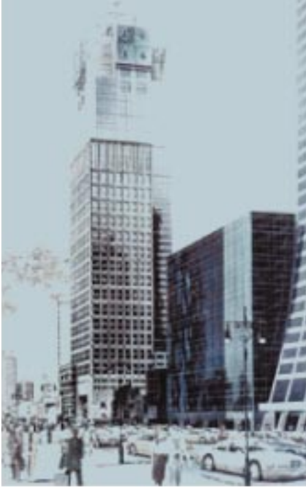
4 Times Square in New York City is one of the first office buildings in the U.S. to be powered by a 200 kW phosphoric acid fuel cell system (Courtesy: International Fuel Cells)
