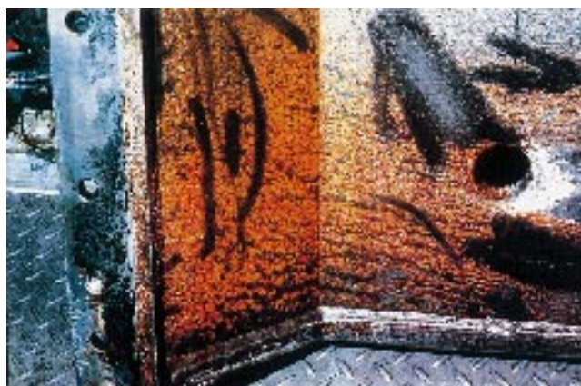
Figure 4.6 Gearbox system which continued to be re-infected until manually cleaned
