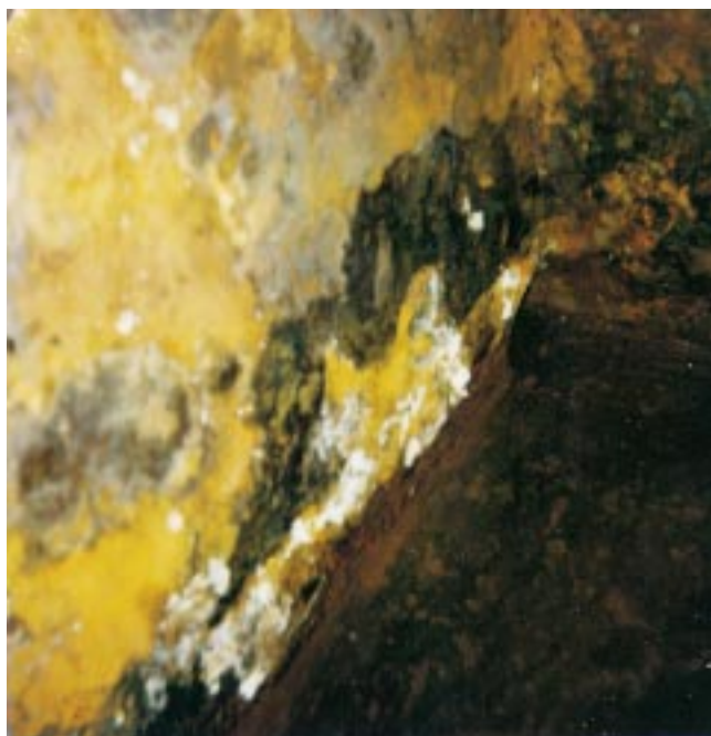
Figure 6.3 Ballast tank corrosion by SRB due to fish oil protection coating before cleaning
