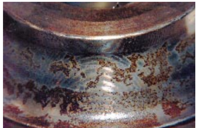
Figure 3.11 Machinery corrosion and oil system contamination from tank top water ingress
