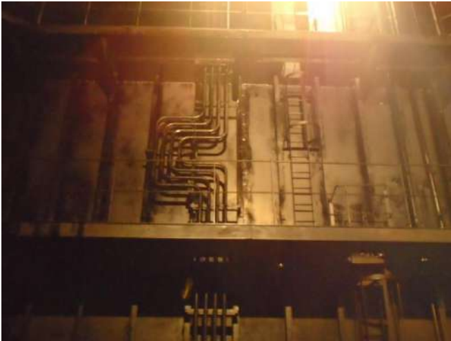
1. Tank sidewall (From the bottom)
